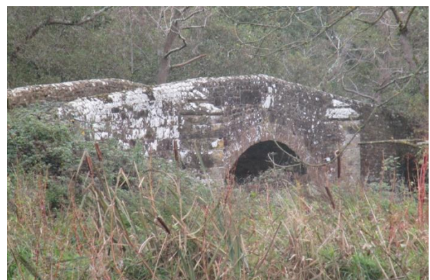
Stone bridge over the River Rother.
